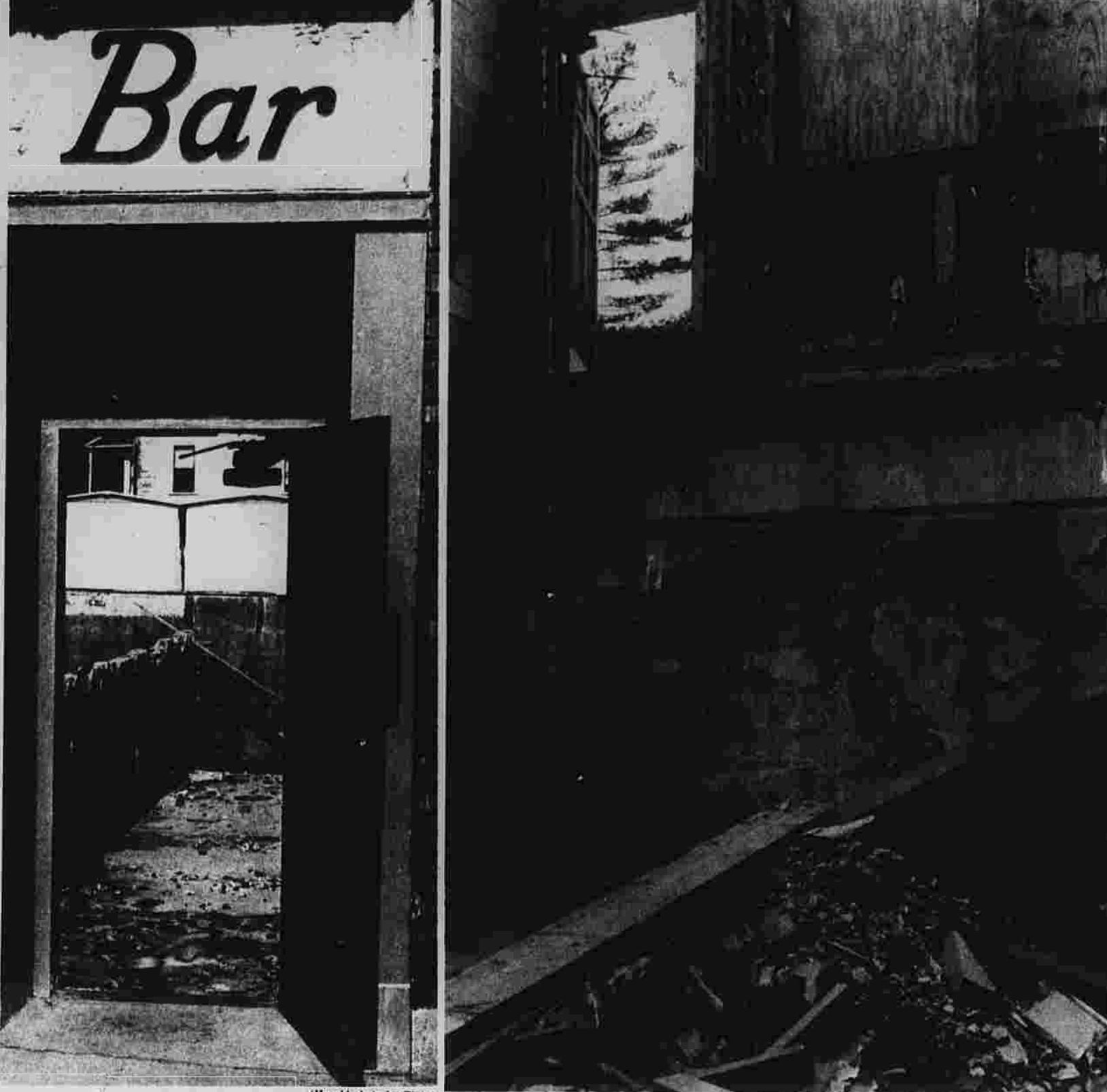
A Condition Under Investigation
